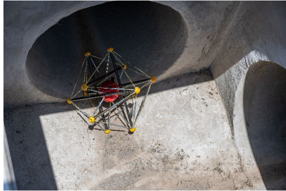
Fig. 7: Tunnel Access Point
