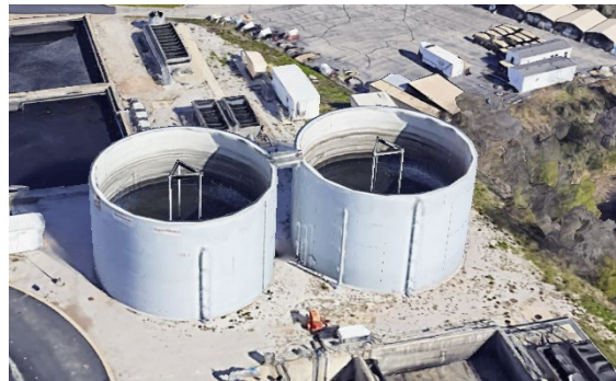
Fig. 5: Simulated Chemical Storage Facility
