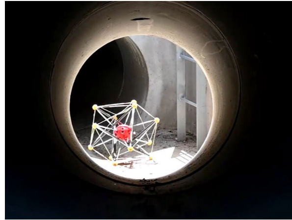
Fig. 26: 4-Gas PLUS sensor deployed in subterranean tunnel
