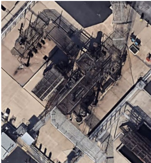
Fig. 13: Petro/Chemical Testing Prop
