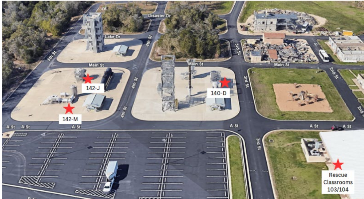
Figure 10: Props used in test Total Safety Monitoring System Service
